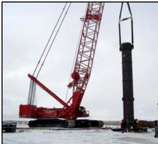
Lowering 6 ft dia. liners with 450 ton crane - Bridger Coal
